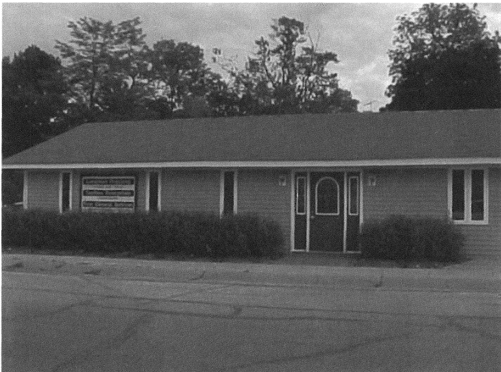
2001 Lake Crest Plumbing.
