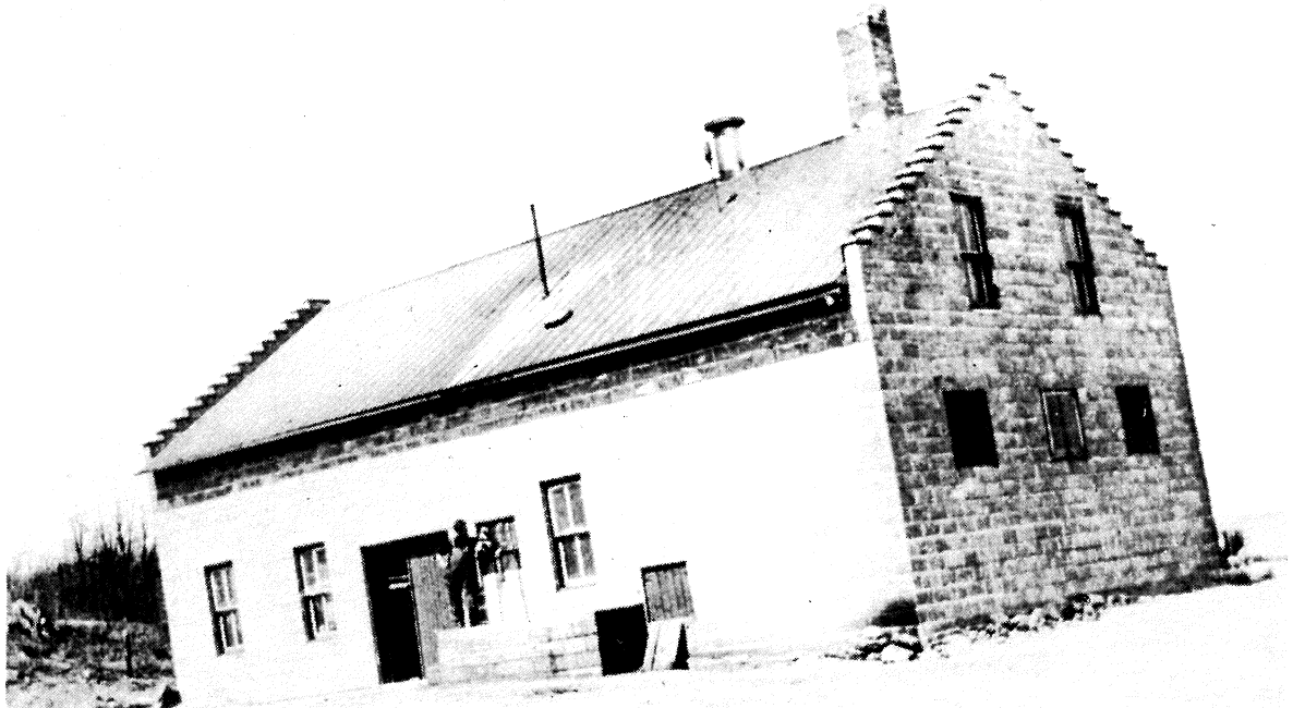
Photo No. 17 - High Street Creamery - About 1913
