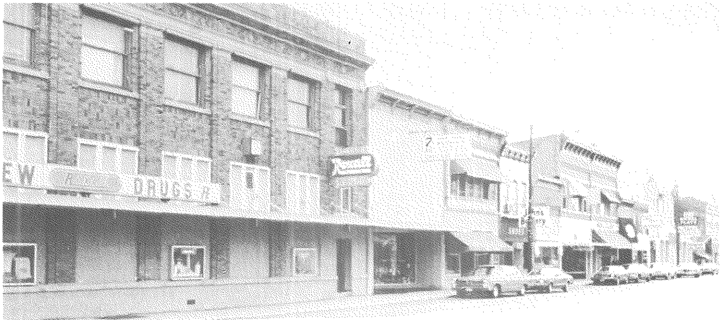
RENOVATED STORE FRONTS greeted visitors to downtown Elkhorn in the fall of 1976. Businesses along South Wisconsin street included Park View Drugs and liquor store, Wolf Jewelry,
