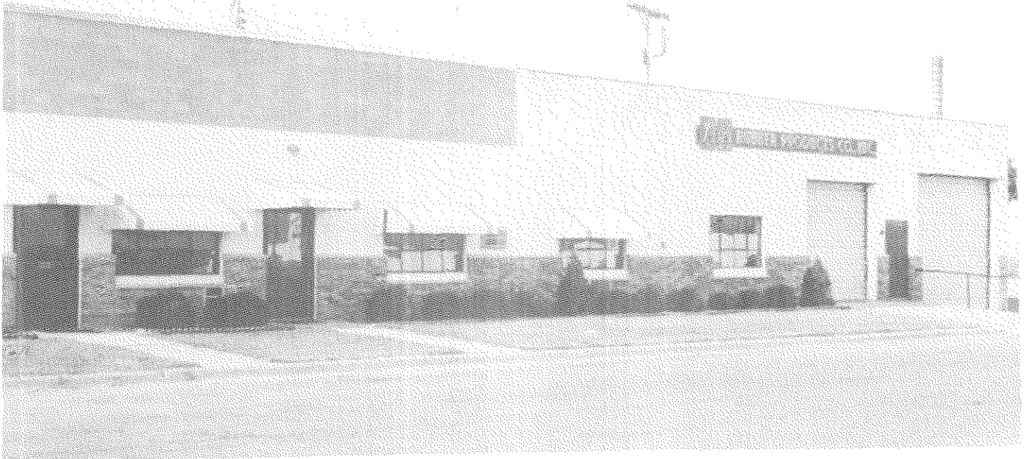
A-K RUBBER PRODUCTS CO. PLANT
