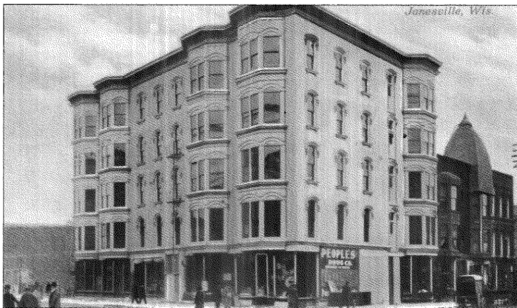
Timothy Jackman built the Jackman Block in 1861. In 1901, a fifth floor was added for Valentine's School of Telegraphy, with four bays along Milwaukee Street and one along North Main Street. After the Jackman family sold the building in 1962, the top two floors and the bays were removed, and porcelainized steel siding was added. In 2001, the building was remodeled again and given another new look. (Adler collection.)
