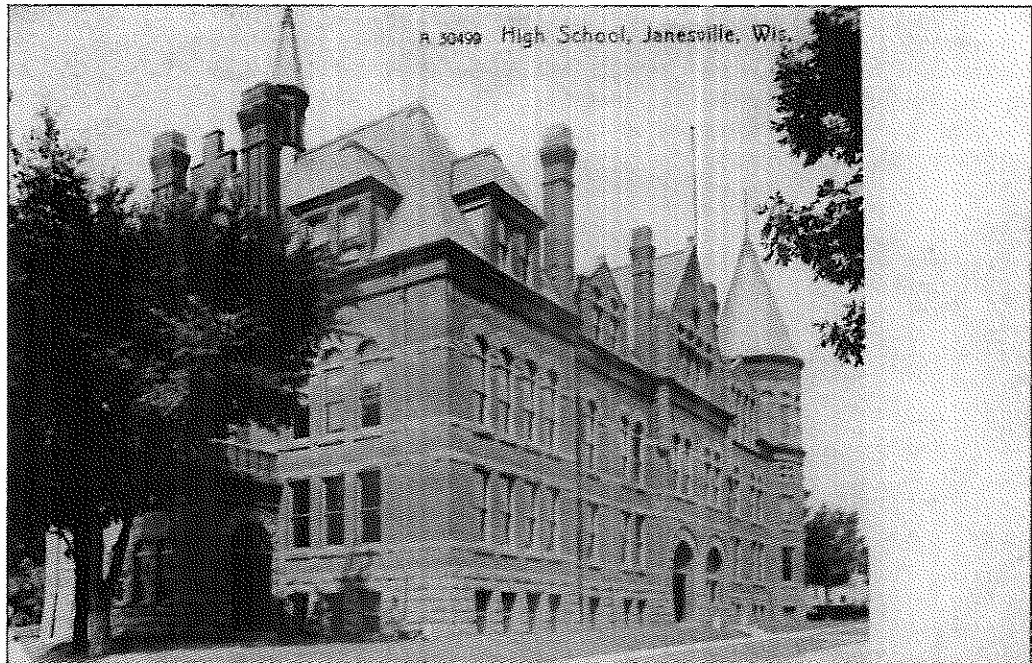
The 1895 high school was designed by W. A. Holbrook of Milwaukee and built by Clark and Stuart. H. C. Buell, the superintendent of Janesville schools, wrote in Brown's 1908 History of Rock County , "In the fall of 1895, the school was moved to the present commodious high school building on High Street." The $56,000, three-story building was constructed of Menominee red pressed brick with red Portage sandstone trim. (Adler collection.)
