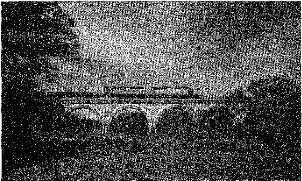
The 1869 stone arch bridge on the former Chicago and North Western line south of Janesville has five 50-foot arches. When heavier diesel locomotives replaced steam engines in the 1930s, the arches were reinforced with steel rods covered in concrete. The bridge is at Tiffany, formerly Shopiere Station, on the Union Pacific's Janesville to Chicago line and can be seen from Smith Road east of the village. (Adler collection.)
