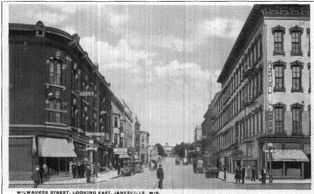
The Smith Block and the Myers Hotel frame this view of East Milwaukee Street. Just past the London Hotel's corner tower on the left is the doorway of the three-story 1880 Hodge and Buchholz Carriage Factory (still extant). Robert Hodge and Herman Buchholz changed the name to the Janesville Carriage Company and built omnibuses, buggies, phaetons, carryalls, sleighs, and circus wagons, selling out to Samson Tractor in 1919. (Dommershausen collection.)
