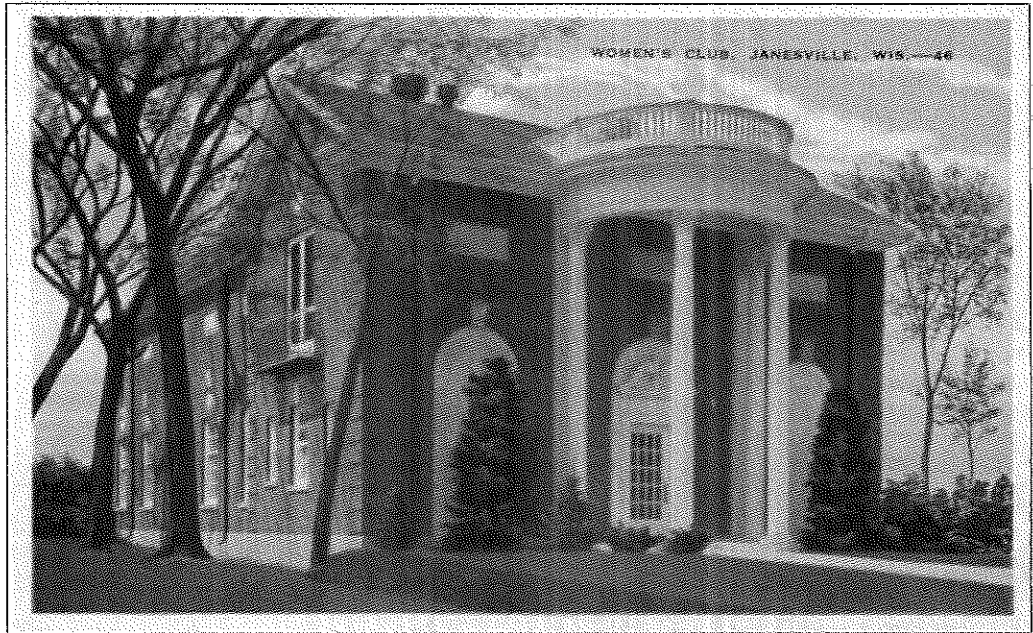
The Janesville Woman's (not Women's as printed on this card) Club Association began in 1927, and a year later this building, still in use, was completed at 108 South Jackson Street. The original plan was to build a gallery for the Women's Art League, but donations and fund-raising led to this larger building that became a meeting place for women's groups in the city. (Adler collection.)
