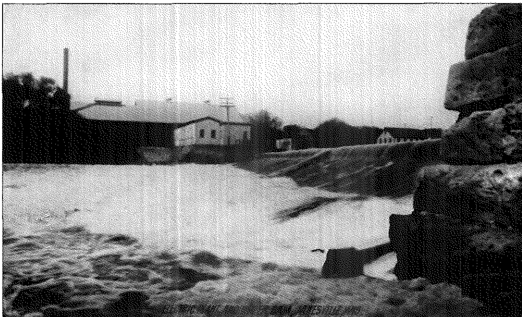
Around 1905, the Rotograph Company published this creative view of the upper dam showing the heavy stonework and the old Janesville Electric Company plant. In 1902, several Janesville businessmen bought this plant from Pliny Norcross and expanded and modernized service in the city. In 1915, they built another hydroelectric plant near the west end of the dam. Part of that plant is still extant. (Adler collection.)
