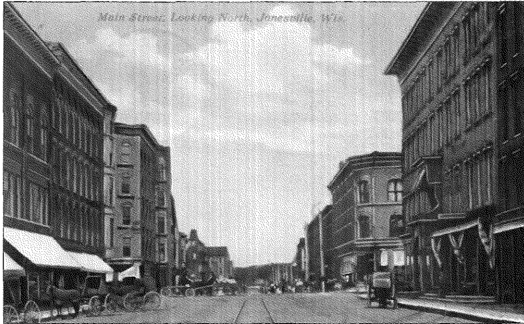
The 1855 Lappin-Hayes Block, to the left, is the only one remaining of the four business blocks that surrounded the Main and Milwaukee Streets intersection. In 1899, Dennis and Michael Hayes bought the Lappin Block. They gutted the interior and installed an elevator and a central light well, as well as a metal cornice and two pressed-metal rounded bays at the corners. It was then renamed the Hayes Block. (Adler collection.)
