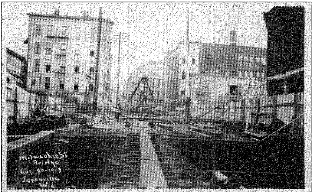
Four months after the fire, repairs were being made. During the night of the fire, flames rose so high that birds miles away could be seen. The fire destroyed the Milwaukee Street Bridge and eight businesses on it. All were made of wood, and two years earlier the state fire marshal warned that Janesville's business district was susceptible to fire. The new bridge was built of concrete; it is still in use. (RCHS collection.)
