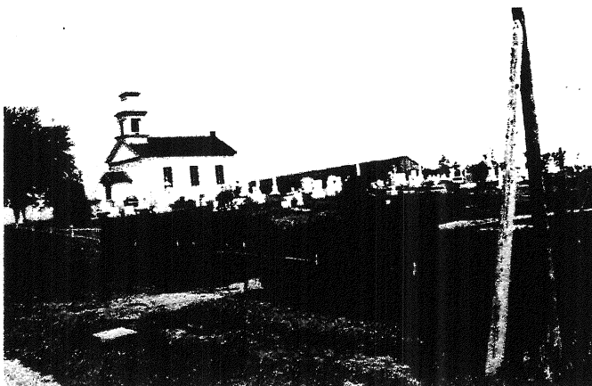
Bristol-Paris Church and Cemetery Note the addition of an entry to the church
