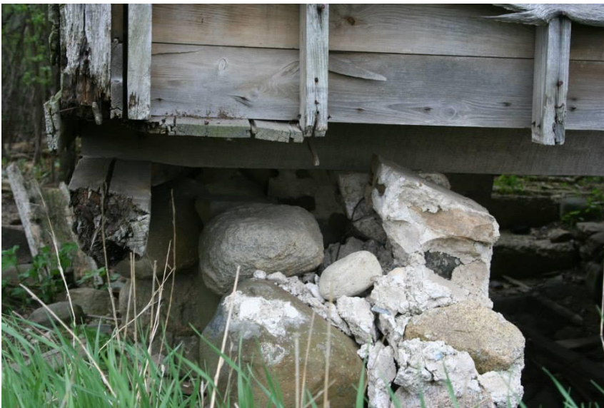
Hilbert house, west side
