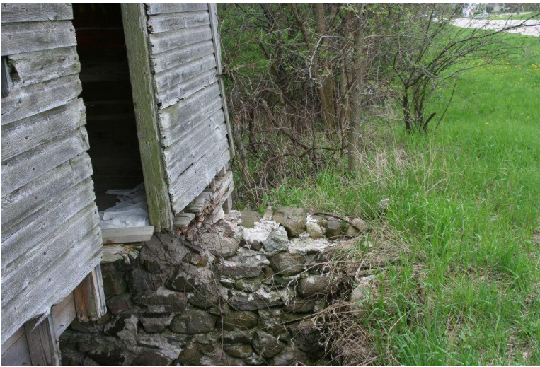
this shows the walls of the foundation.
