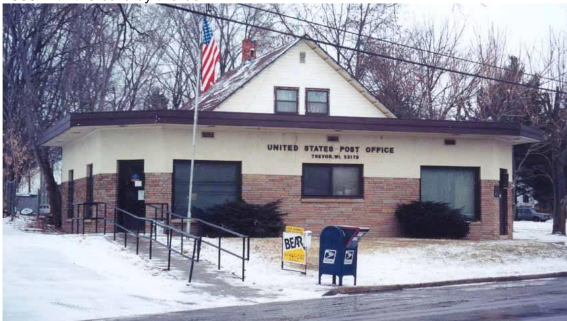
2006 with the curb by the box - this area has since been changed to be a slope.
