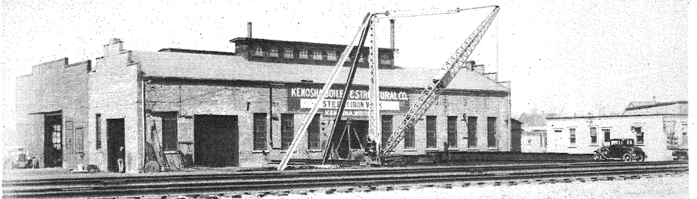
Kenosha Boiler and Structural Co. began in this building 71 years ago committed to service, quality and customer satisfaction.
