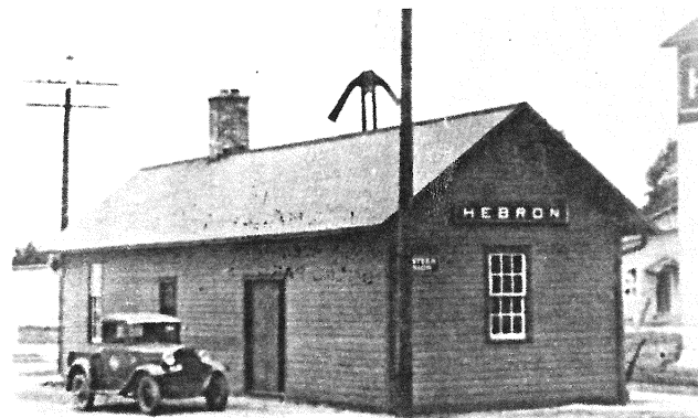
Above: upper, the rear of Capron depot. Lower, east end and rear of Hebron depot. Note the old pickup truck used for Railway Express deliveries. Facing page: three views of Pleasant Prairie depot. Upper, looking west. Middle, when this photo was taken, Pleasant Prairie, like some other KD depots had been closed for several years. Lower, west end and rear. All photos taken in August, 1938 by James Penhallegon, courtesy Bill Armstrong.
